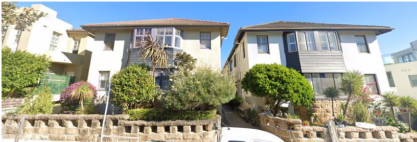
Figure 67: 127-129 Hastings Parade, North Bondi (Source: Google Maps Street View, November 2023)
