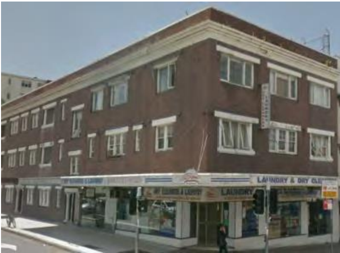
Figure 6: View of 160 Bondi Road, Bondi (Source: Draft Heritage Data Form, Waverley Council, p.7)
